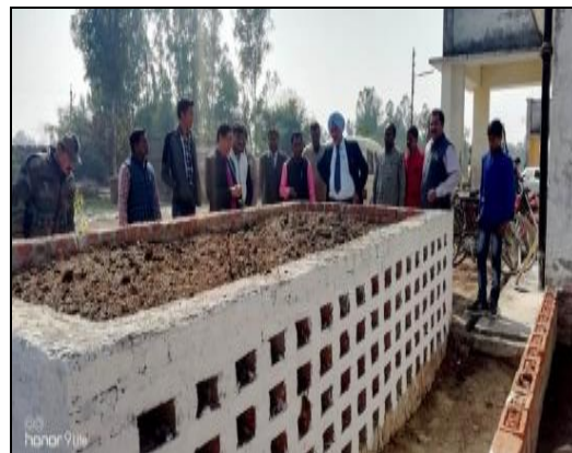
2- NADEP Compost Unit
